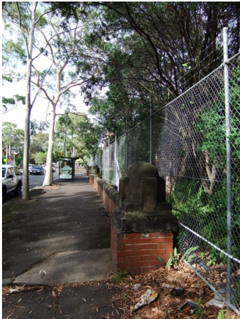
Figure 12 – Historic wall on Joynton Ave
